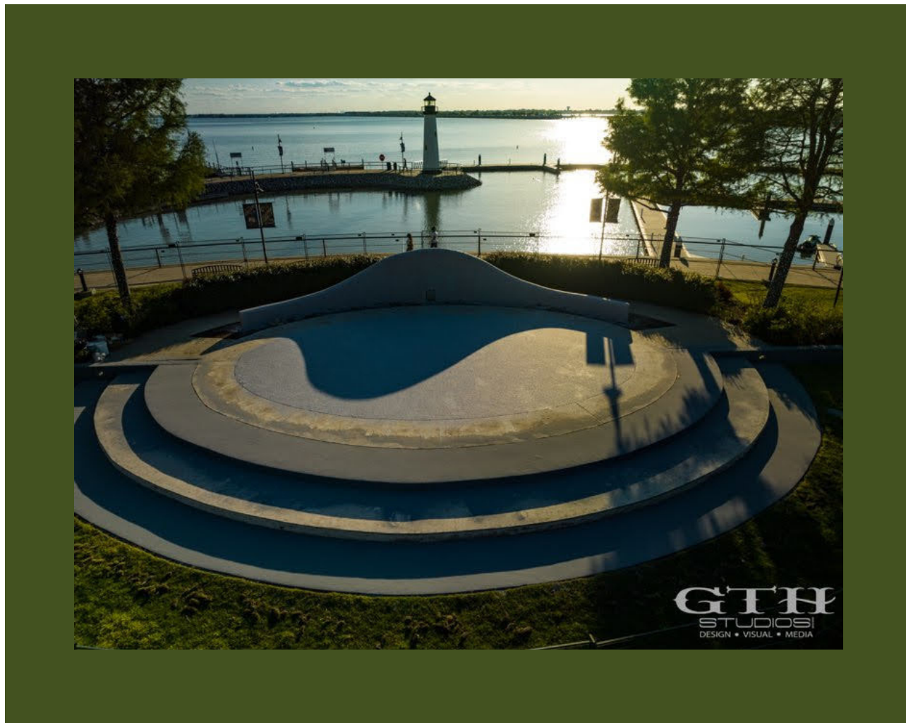
AMPHITHEATER EPOXY PROJECT
